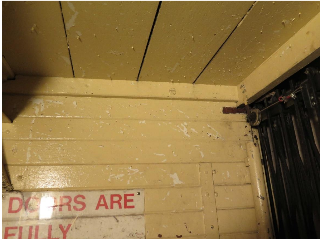
Figure 10 – Detail of the goods lift car showing the junction of the timber panel walls and ceiling and the opening mechanism of the metal scissor doors (Source: NBRS+PARTNERS, October 2015)
