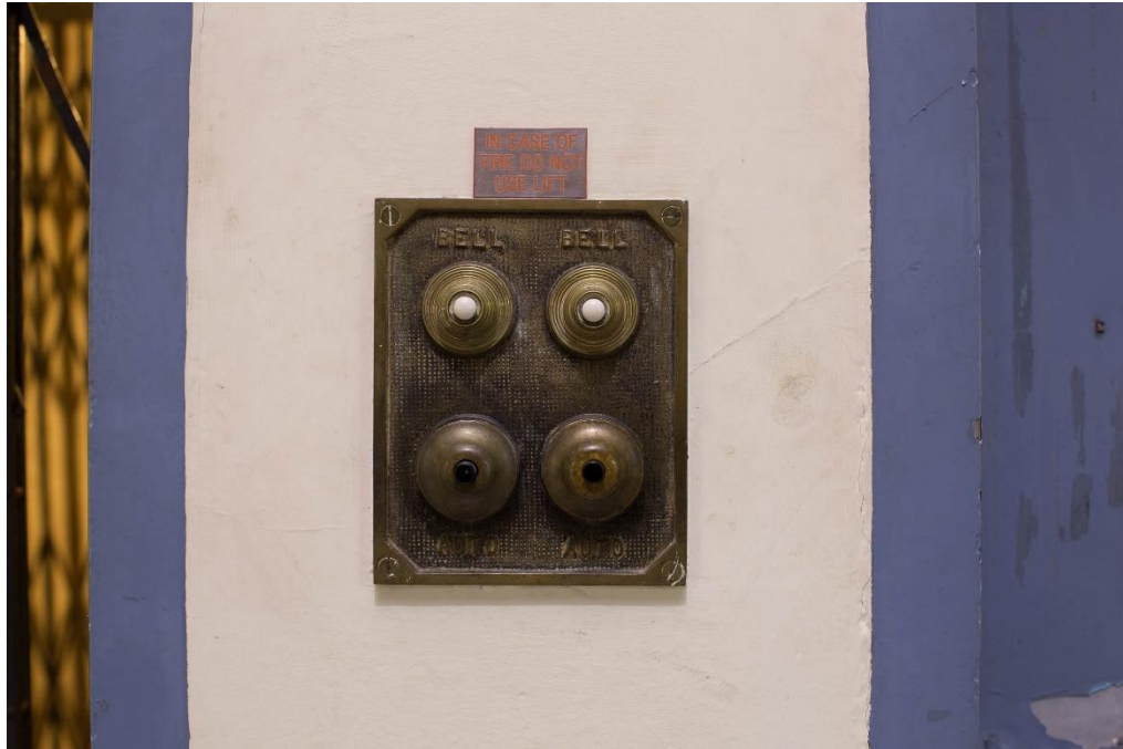
Figure 20 – Dymocks Building, Goods Lift, Wall Between Goods Lift Cars showing brass indicator panel and button press (Source: Alexander Mayes Photography, 2016)
