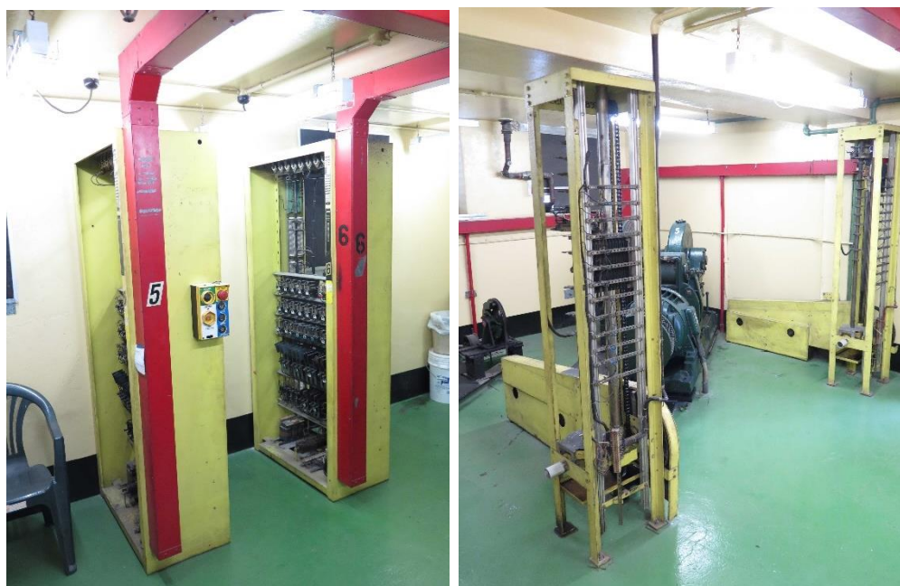
Figure 13 — Roof Level, showing view to Otis goods lift equipment including winches and switches in the Motor Room (Source: NBRS+PARTNERS, October 2015)
