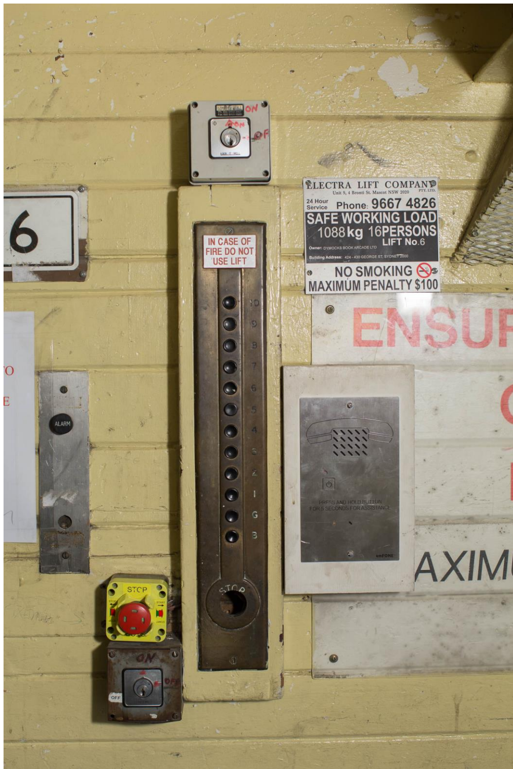
Figure 19 – Dymocks Building, Goods Lift, Interior of Car – showing the indicator panel and button press (Source: Alexander Mayes Photography, 2016)
