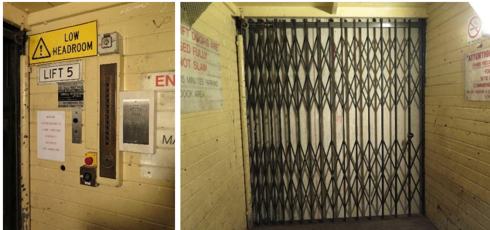
Figure 9 — The interior walls and ceilings of the goods lift car are lined in timber panelling and painted. The original button press panel is located on the wall of each car. The metal horizontally-opening scissor doors are located at the eastern and western door openings. (Source: NBRSPARTNERS, October 2015)
