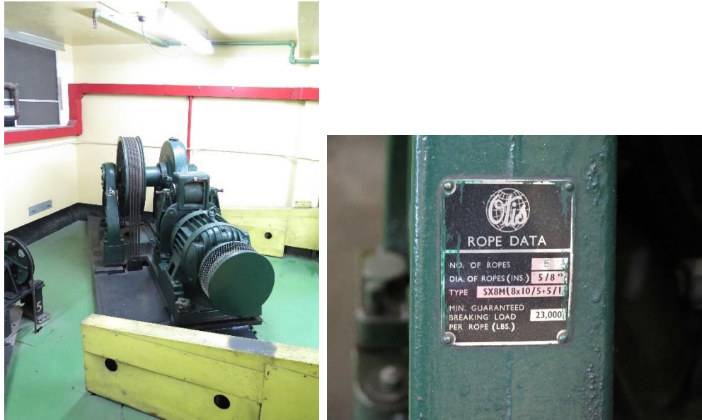
Figure 14 – Roof Level, showing view to Otis goods lift equipment, including winches and switches, in the Motor Room (Source: NBRS+PARTNERS, October 2015)
